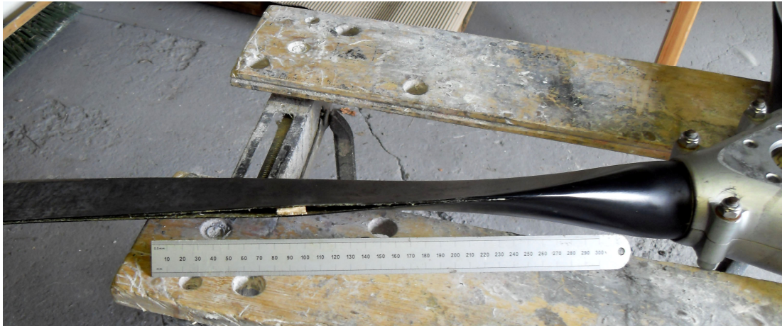
Figure 2 – delaminated trailing edge
