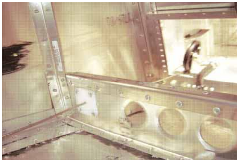
Figure 4 – View of port fuselage wall, looking forward
