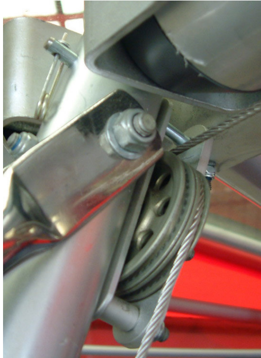
Figure 5; replacement pin above pulleys.
